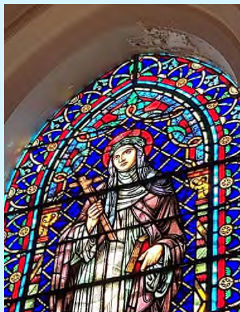
Stain Glass Windows and Caulking
