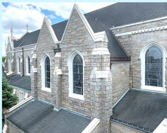
Flashing and Lower Roof
