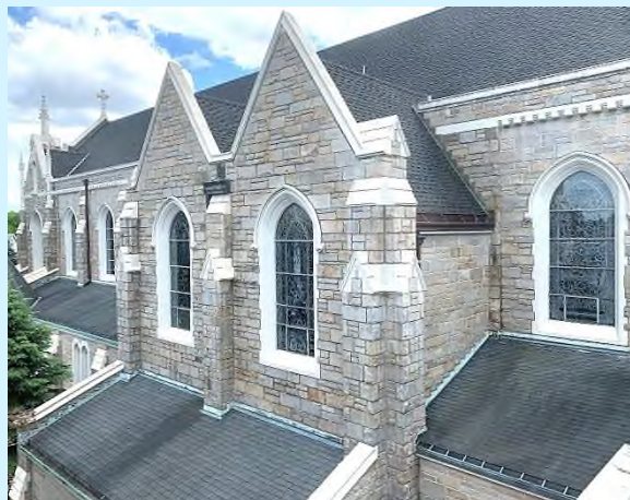
Flashing and Lower Roof
