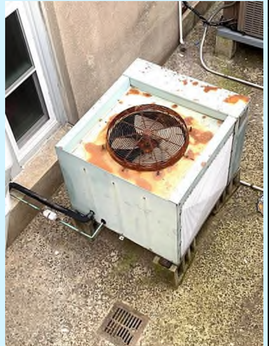
Replacing AC Unit
