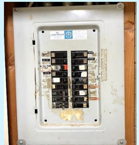
Electrical Service and Panel Upgrades
