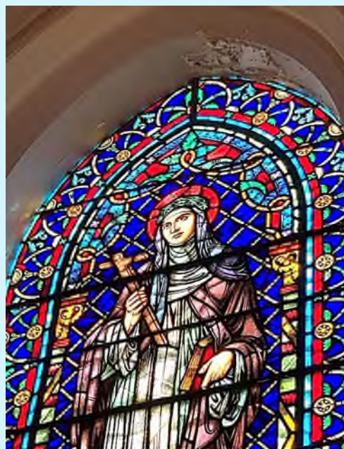
Stain Glass Windows and Caulking
