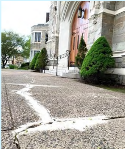
Replace Concrete Walkways in front of the Church
