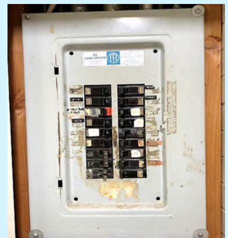
Electrical Service and Panel Upgrades
