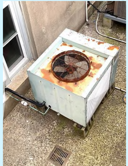
Replacing AC Unit
