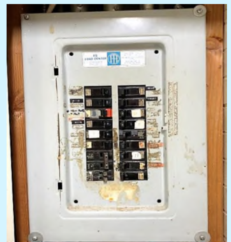
Electrical Service and Panel Upgrades
