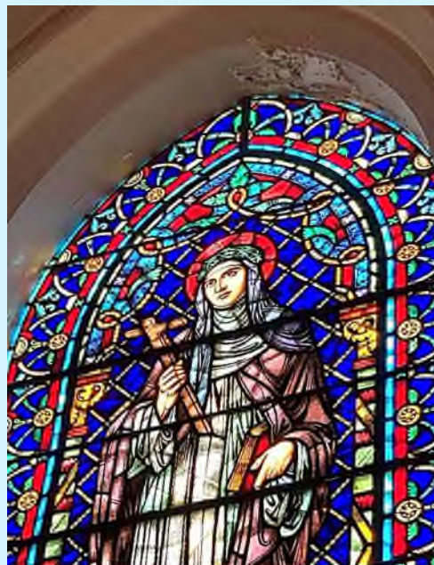
Stain Glass Windows and Caulking
