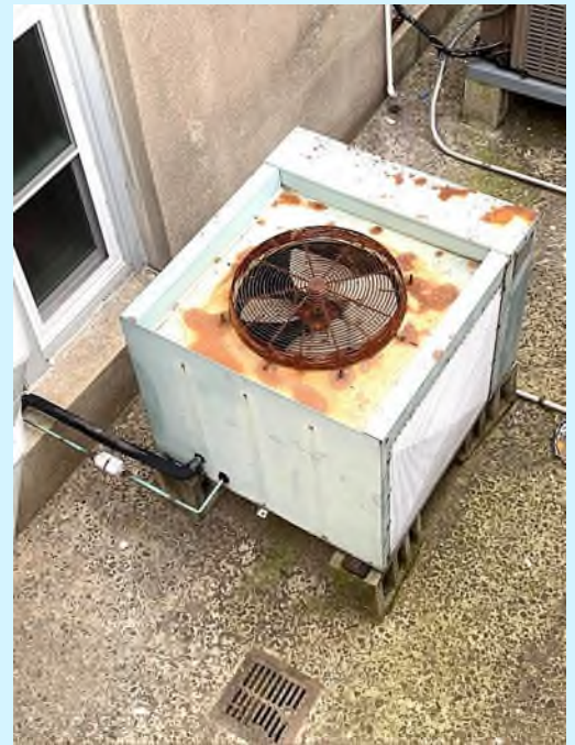
Replacing AC Unit
