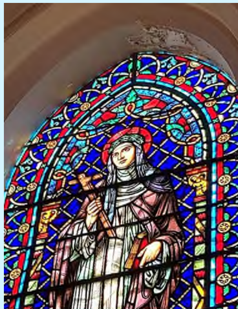
Stain Glass Windows and Caulking
