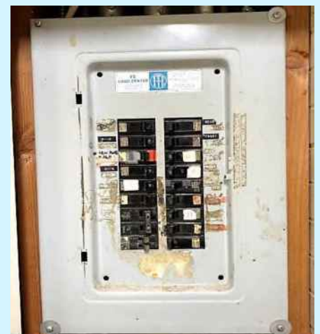
Electrical Service and Panel Upgrades
