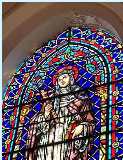
Stain Glass Windows and Caulking
