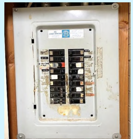
Electrical Service and Panel Upgrades
