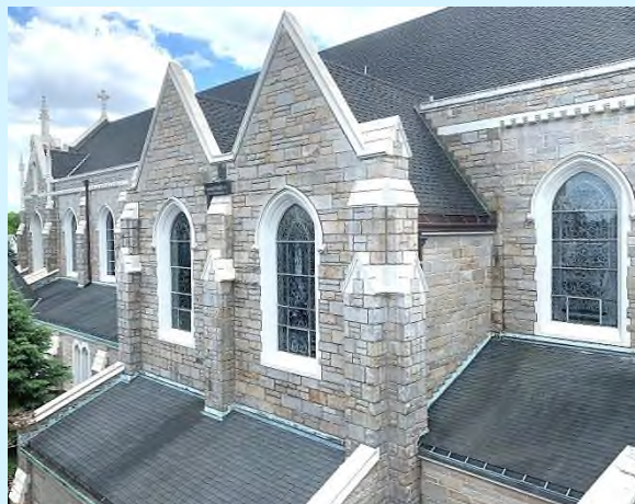
Flashing and Lower Roof
