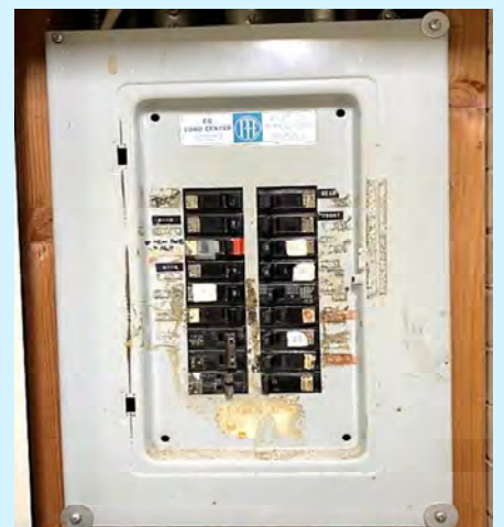
Electrical Service and Panel Upgrades
