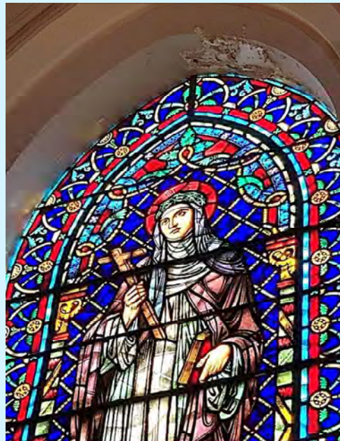
Stain Glass Windows and Caulking
