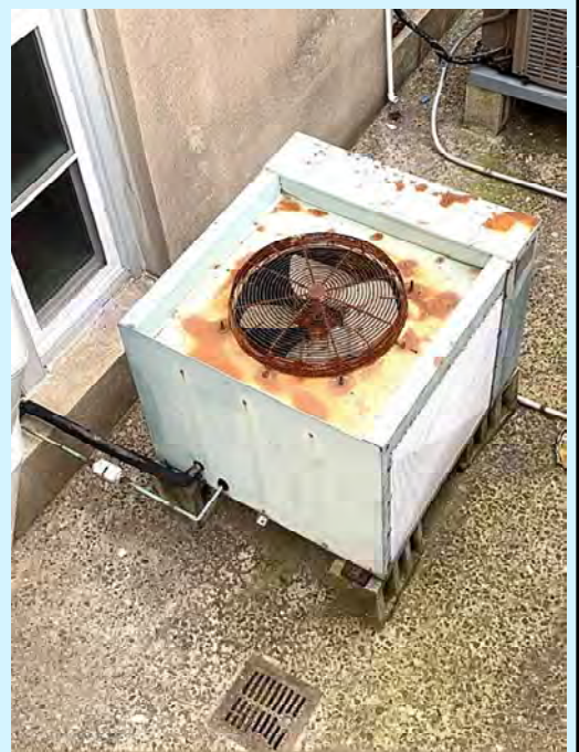
Replacing AC Unit
