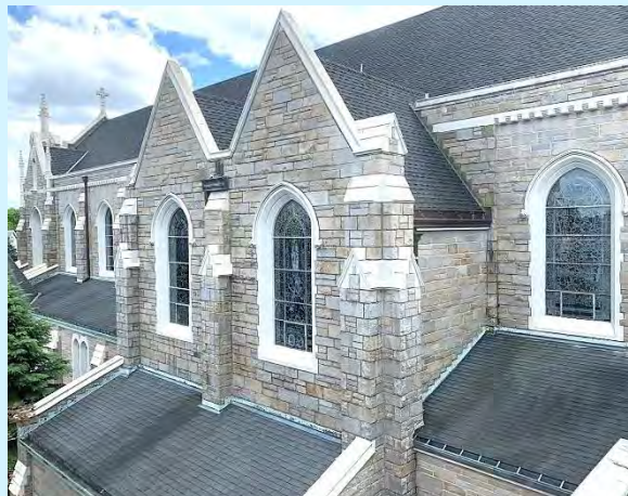
Flashing and Lower Roof
